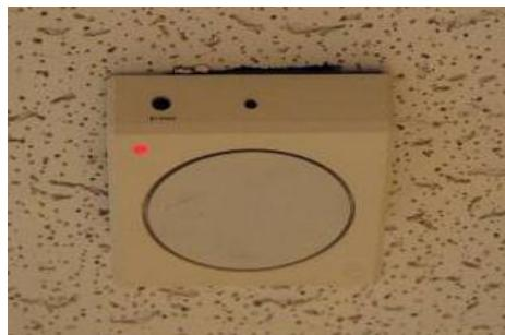
**Figure 6: Motion sensor to turn lights on/off**
