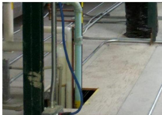
**Figure 4: Wood insert within floor of interstitial space**
