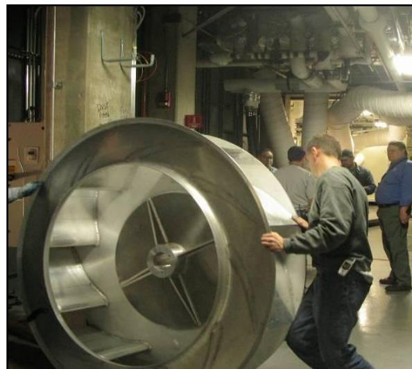
**Figure 13: Replacing the fan within the 68,000 CFM air handler**
