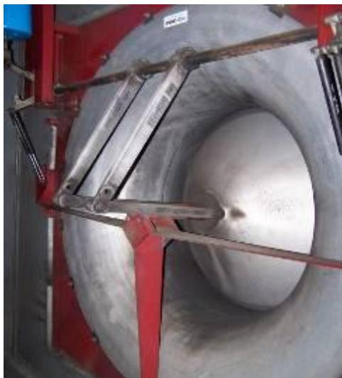
**Figure 12: Econo-cone within the 68,000 CFM air handler**
