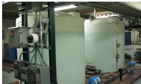
**Figure 9: Cage pre-wash water storage tanks**
