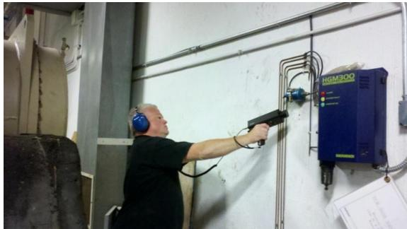
**Figure 8: Using an ultrasonic handheld device to look for leaks in pneumatic control lines**
