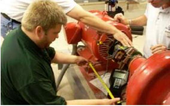
**Figure 4: Laser alignment of a pump**
