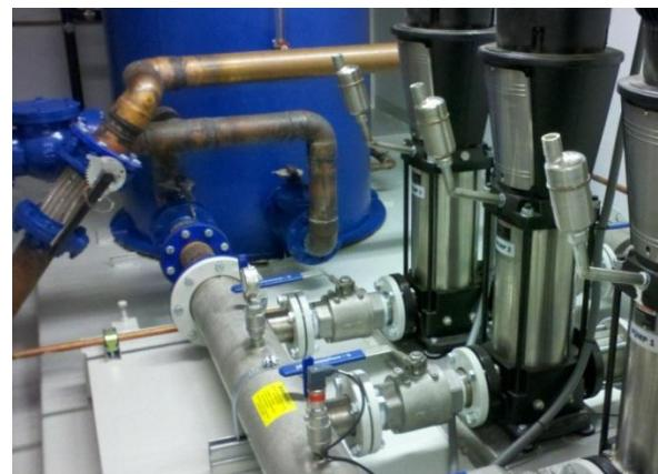
**Figure 4: Domestic water pressure station**
