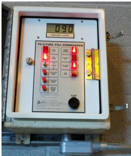
**Figure 1: Enclosure with generator fuel indicators**
