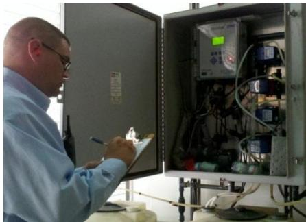
**Figure 2: Utility engineer checking pH levels of cooling tower water**
