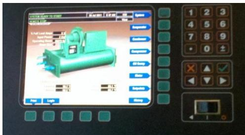
**Figure 3: Chiller control panel**
