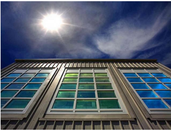
nano-crystal studded glass changes color to filter light
